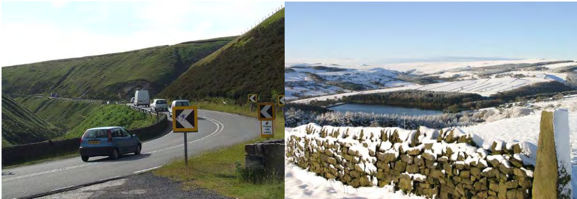
Figure 2-4 Tortuous Road Alignment on Snake Pass and Typical Moorland in the West of SCR
