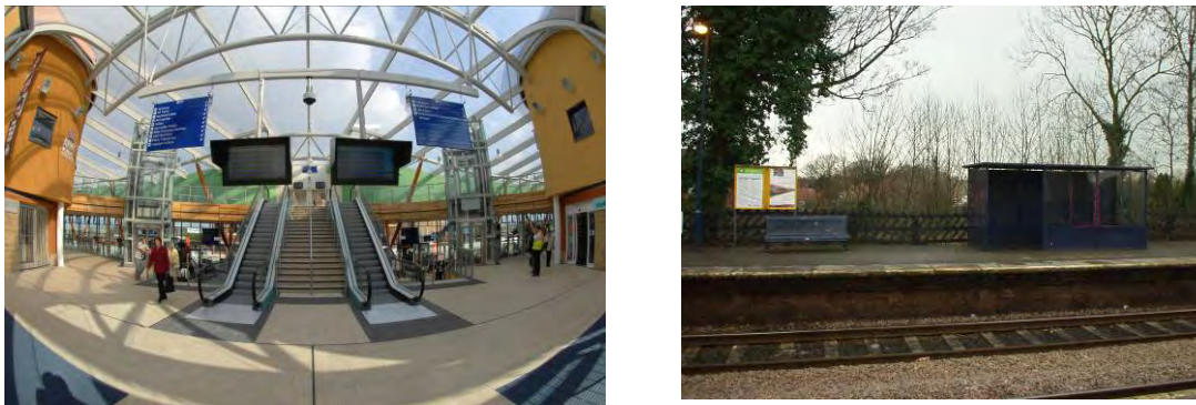
Figure 2-13 Barnsley Interchange and Thorne North Railway Station
